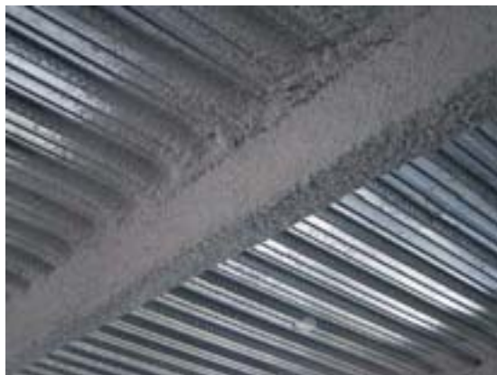
Fig I.1 Beam protected with SFRM.
